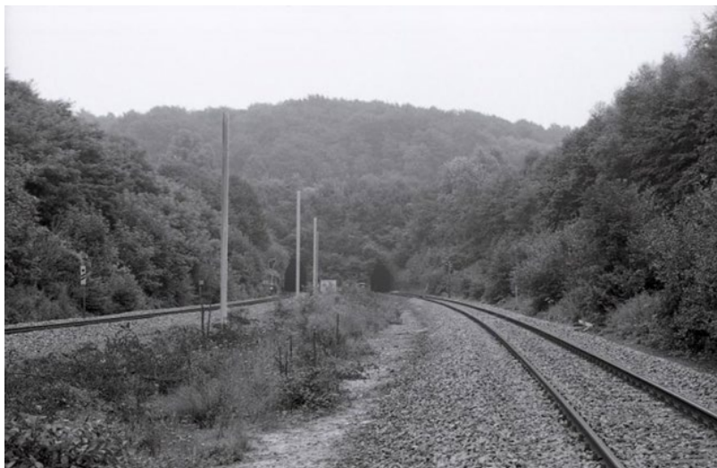
Tunnel in Veurs (Ref: MZ19971)
