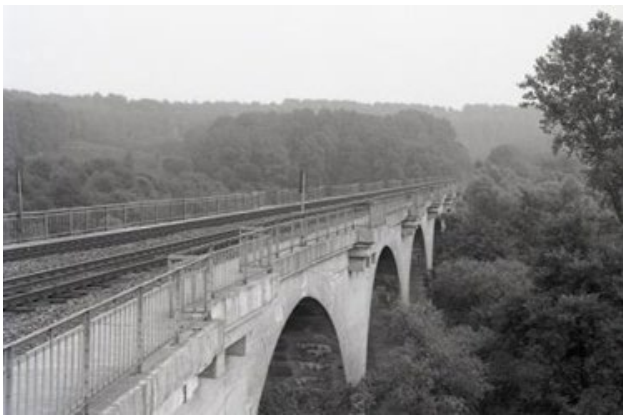
Viaduct van Remersdaal (Ref. MZ20011)
