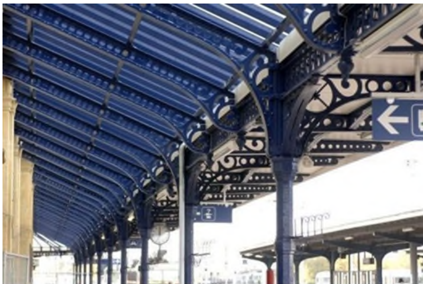
Detail van de luifel na restauratie, 2007 (Ref. D3099-23)
