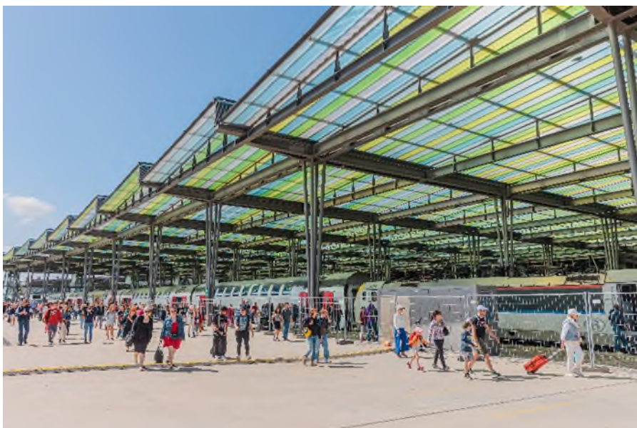
Nieuwe luifel in station Oostende, 2022 (Ref. B0216-25)
