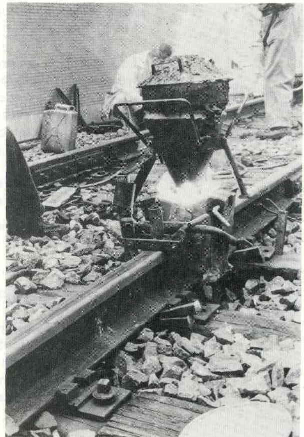
Figure 8.28 Coulée du joint.
