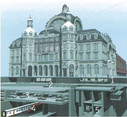
The aboveground Astrid square will be renewed and four underground levels will be created.
