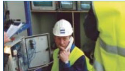
LE POSTE DE PILOTAGE ÉTAIT SITUÉ À ÉGALE DISTANCE DES DEUX AXES DE POUSSAGE. LE PILOTE DISPOSAIT D'ÉCRANS QUI LUI PERMETTAIENT DE CONTRÔLER LA PROGRESSION DE LA STRUCTURE. IL ÉTAIT EN CONTACT PERMANENT AVEC LES OPÉRATEURS AUX DIFFÉRENTS POSTES DE GLISSEMENT ET DE POUSSAGE.
