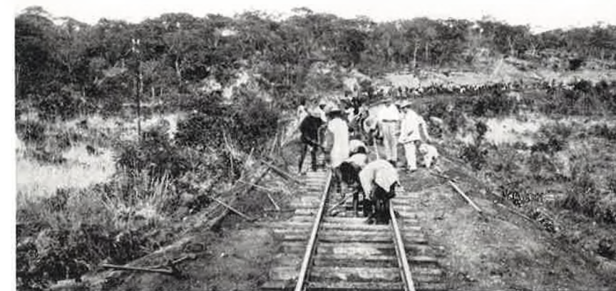
Relaying on the main line, Rhodesia Railways.
