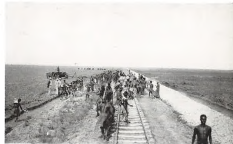
Platelaying across Chifu Maji Plains, Benguella Railway.
