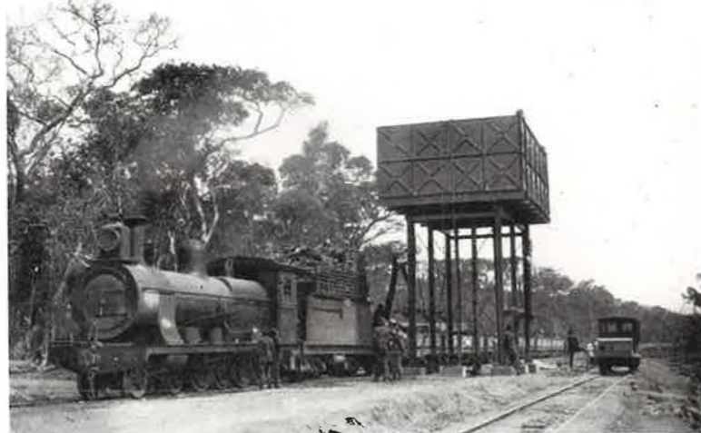
On construction, Benguella Railway.
