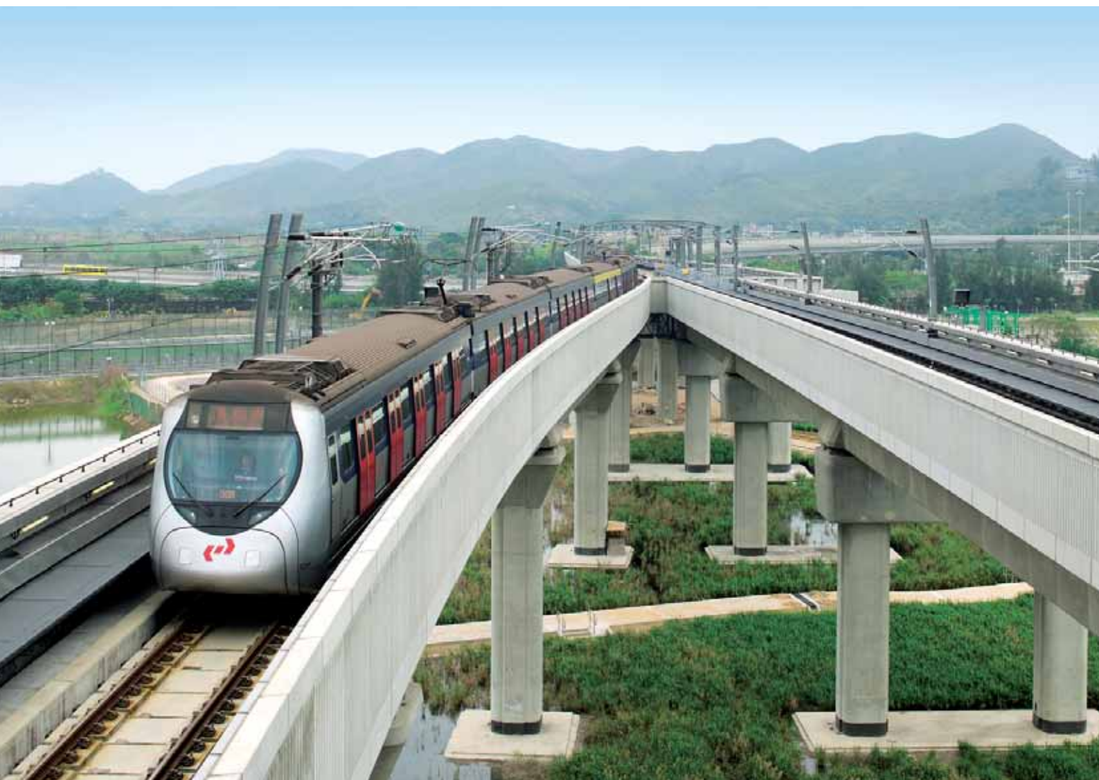
The Lok Ma Chau Spur Line is on track for commissioning in 2007
