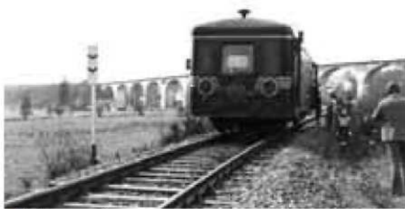
▲ Viaduct van Born
