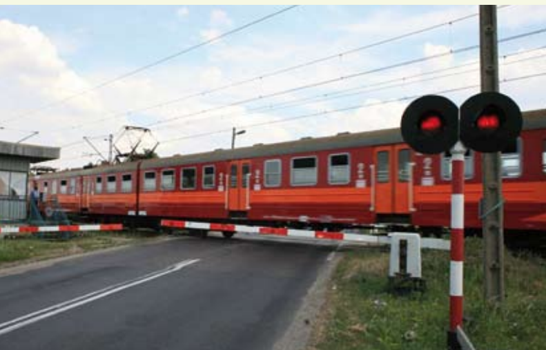
The road rail interface at level crossings presents specific challenges
