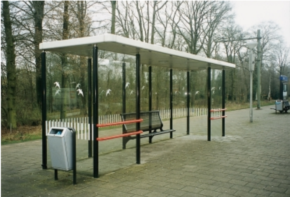
Photo 5.16 Ermelo Station (Netherlands) - waiting shelter
