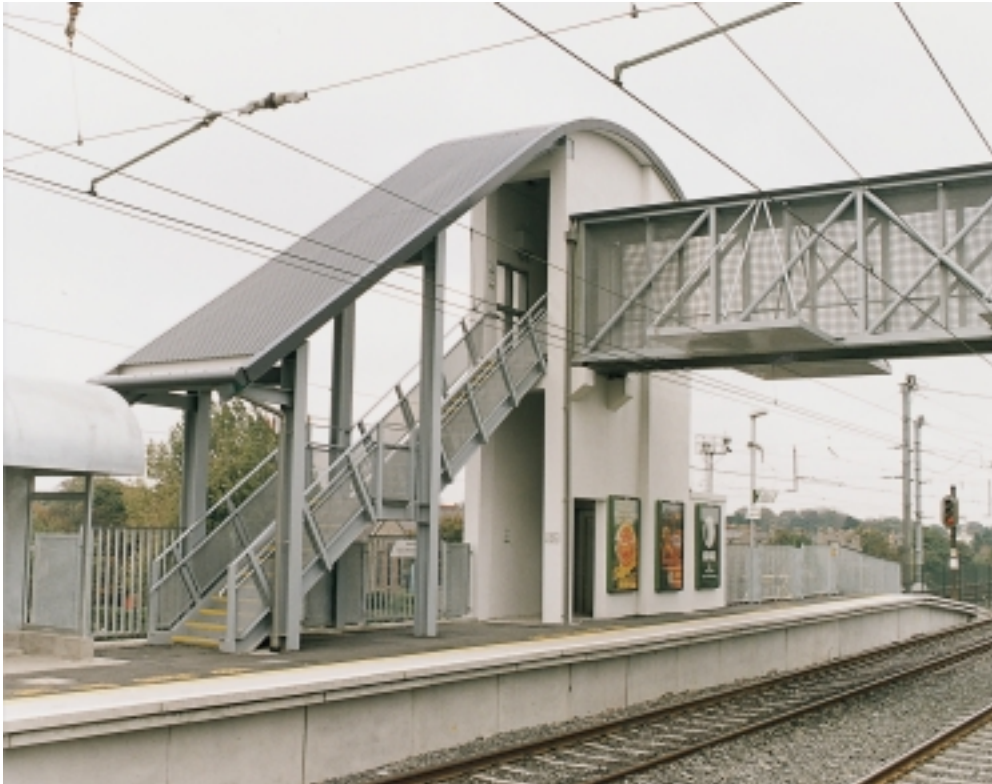
Photo 5.12 Clontarf Road Station (Ireland) - foot bridge
