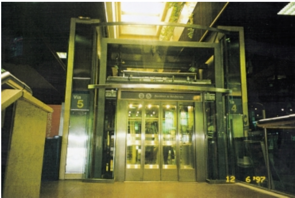
Photo 5.7 Chamartin Station (Spain)
