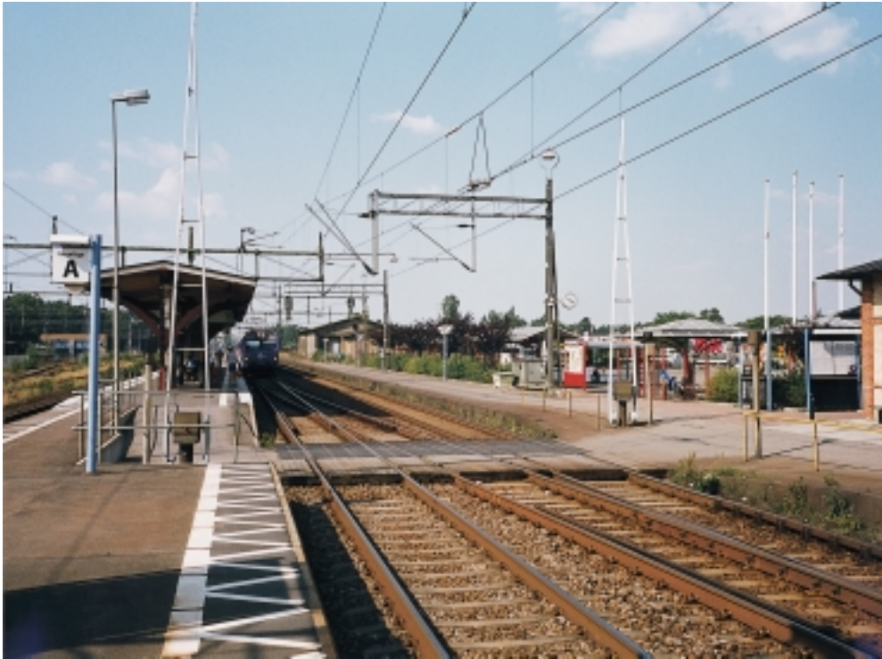
Photo 5.15 Angleholm Station (Sweden) - level crossing
