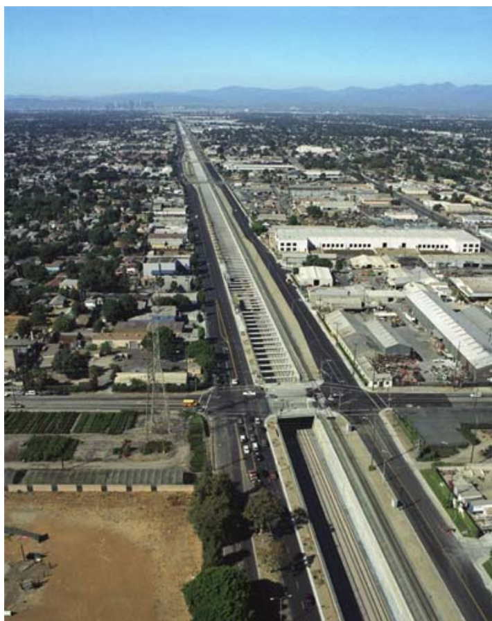
Alameda Corridor (US)
