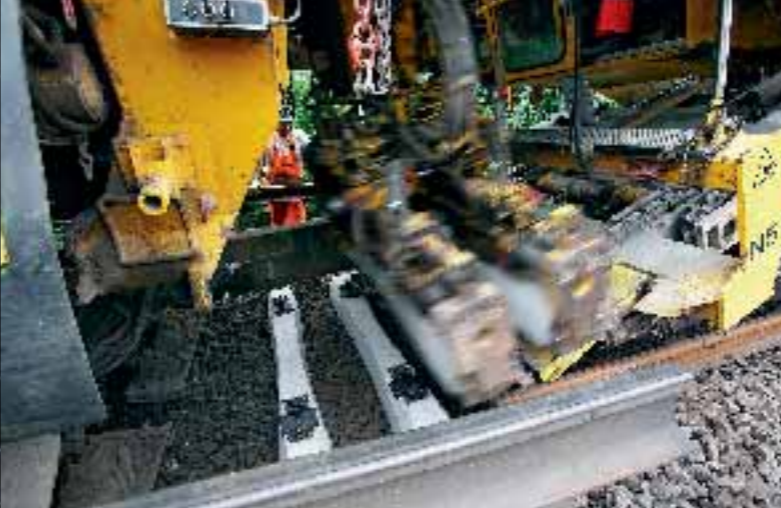
Track bed Bit by bit, a new track appears. View into the cab of the tie laying unit on the track renewal train (below).
