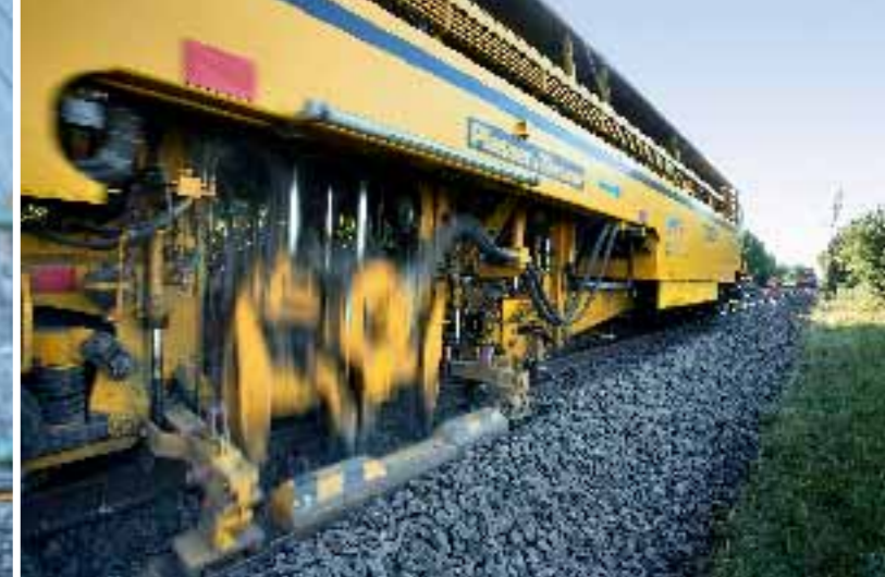
Good, solid work The cleaned ballast is compacted in a series of tamping runs. The spreader (below) helps to thread the new rails into the ties.
