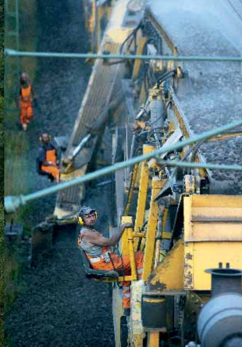
Good, solid work The cleaned ballast is compacted in a series of tamping runs. The spreader (below) helps to thread the new rails into the ties.
