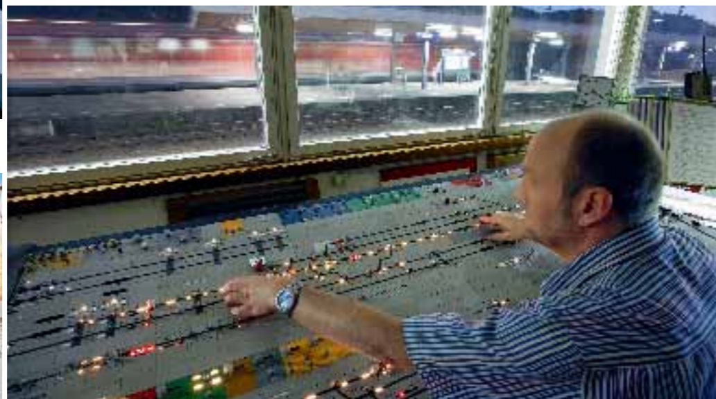
Train management All-relay interlocking is used to control switches and signals at Hausach station.
