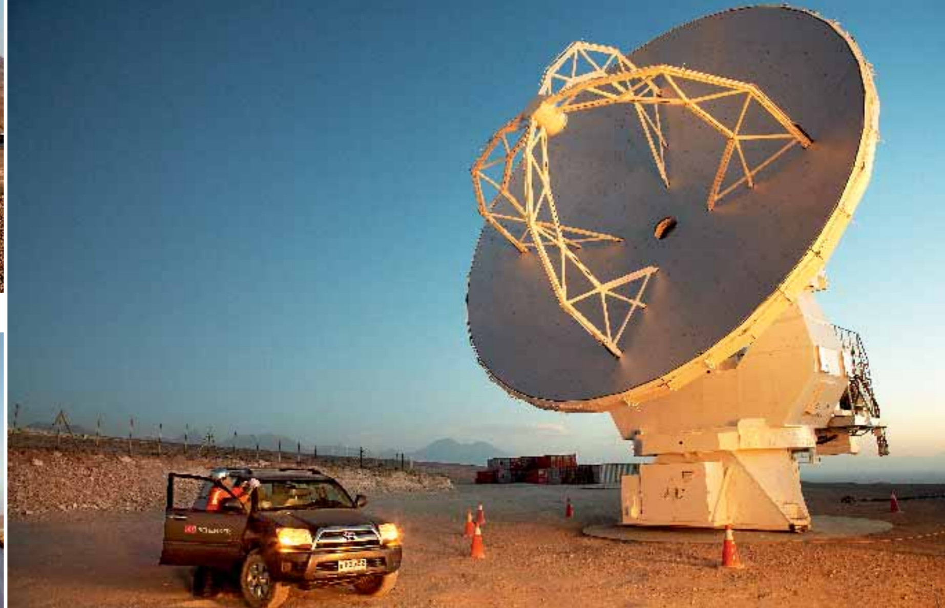
A first peek At 2,900 meters above sea level, the antenna dishes (in this case a Japanese dish, with a diameter of 12 meters) are assembled before being transported to the high plateau.
