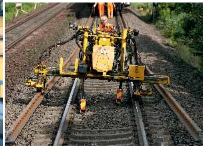
Good, solid work The cleaned ballast is compacted in a series of tamping runs. The spreader (below) helps to thread the new rails into the ties.
