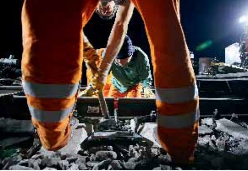
Precision work Once the new rails have been laid, the next step is to align and join the ends.
