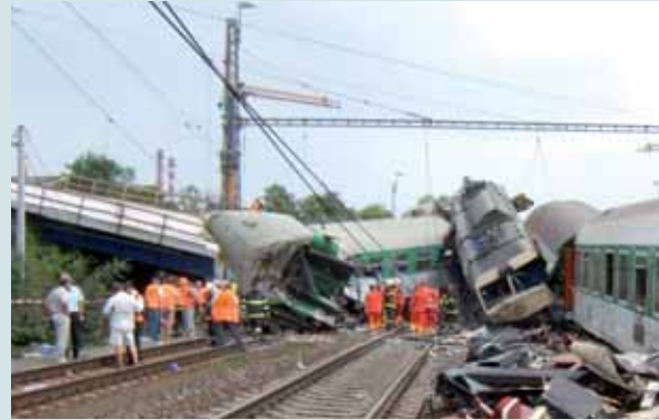
Image 3. Bridge collapse, Czech republic, 8 August 2008. Photo: Czech NIB
