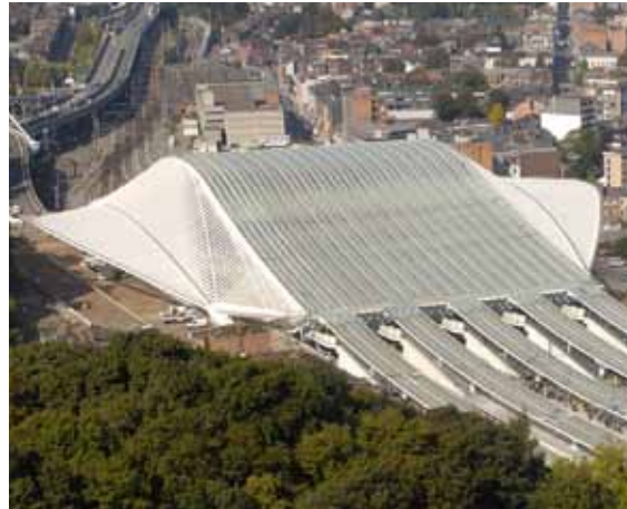
General view of the station from Cointe Hill.
