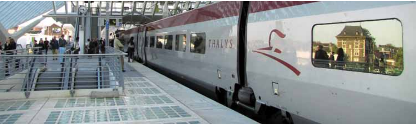
Glass bricks carpet the platforms: the Grande Galerie is lit by natural daylight.
