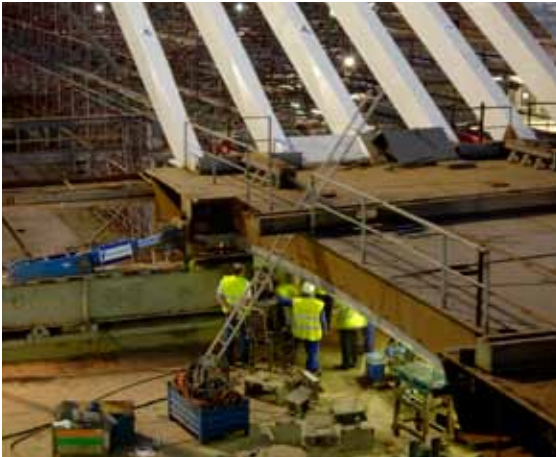
Hydraulic jacks push the arches over the tracks.
