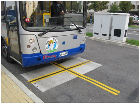
Picture 6-6: Inductively charged electric bus in Turin, Italy.
