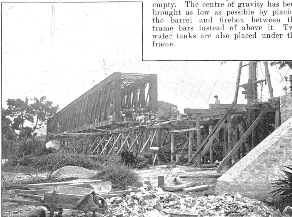
ERECTING BRIDGE TO CARRY THE CONGO RAILWAY ACROSS THE INKISSI RIVER.
