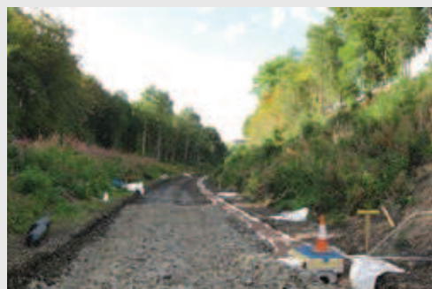
Photo 3.9 Drainage alongside the rail line to prevent flooding
