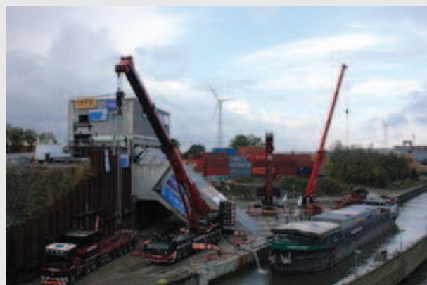
Photo 3.10 Installation of new locks in the Albert Canal © De Scheepvaart
