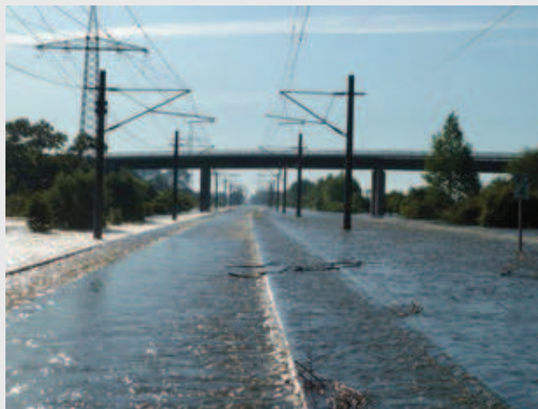
Photo 2.3 Flooding of the Hannover-Berlin railway line
