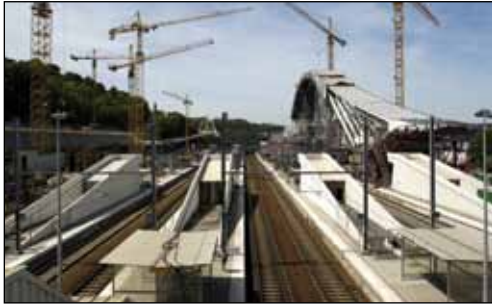
Le chantier de la gare. © SNCB-Holding.
