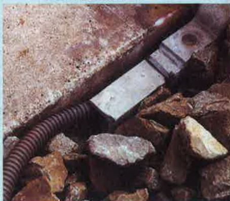
▼ GRONDUTRUSTING IN DETAIL
