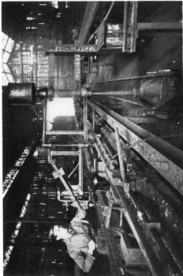
Pneumatic drill, mounted on movable arm, drilling top side rails
