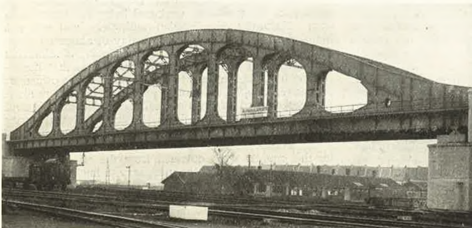
Steel bridge spanning the steam lines to the north of Malines station, Belgian National Railways
