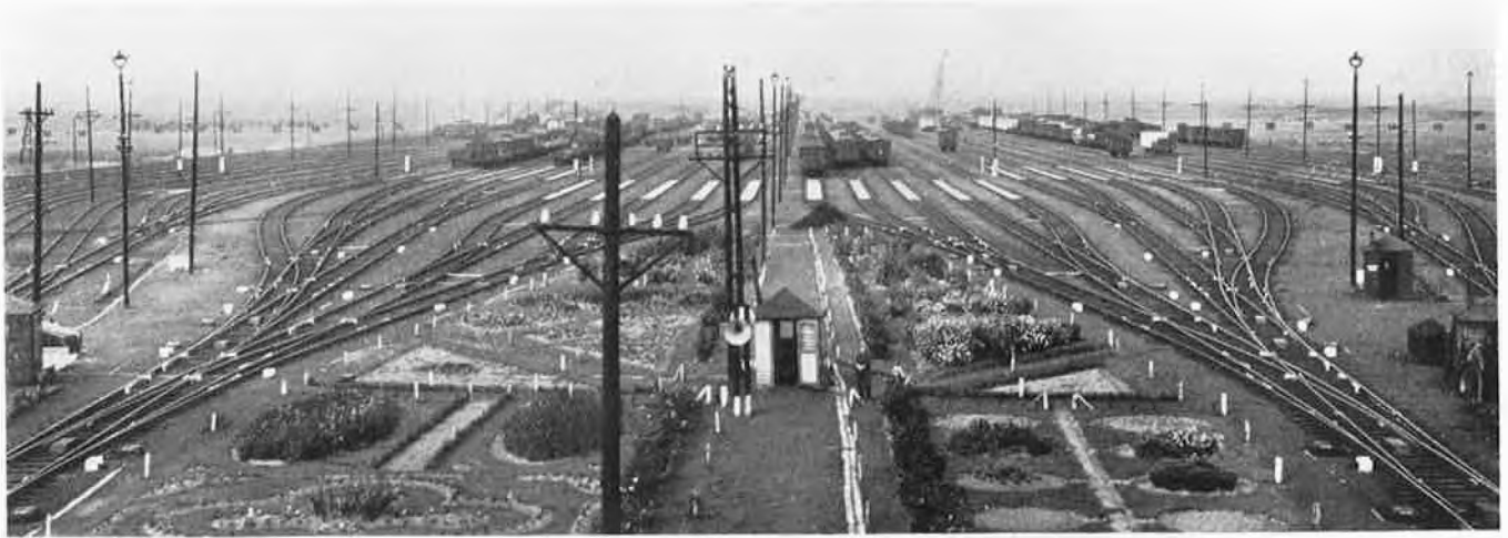
Flower-beds and lawns form an unconventional but attractive foreground to the marshalling yard at Antwerp Nord. Note the loud speakers for transmitting orders to shunters
