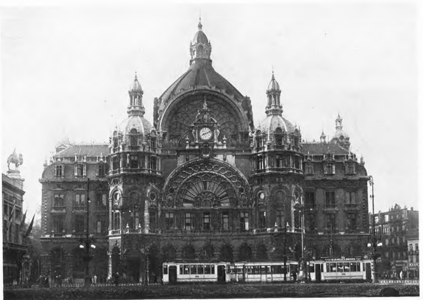
There is an ecclesiastical note in the dome and pinnacles of the Central station at Antwerp which echoes the magnificence of the cathedrals and churches of the city
