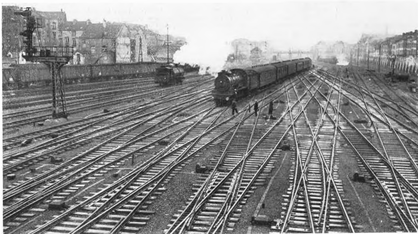
In connection with alterations to the lines at Brussels Nord, Belgian National Railways, to accommodate the trains on the new electrified lines between there and Antwerp, electric signalling has been installed. Above is a view of the approach to Brussels Nord station, showing power-operated points
