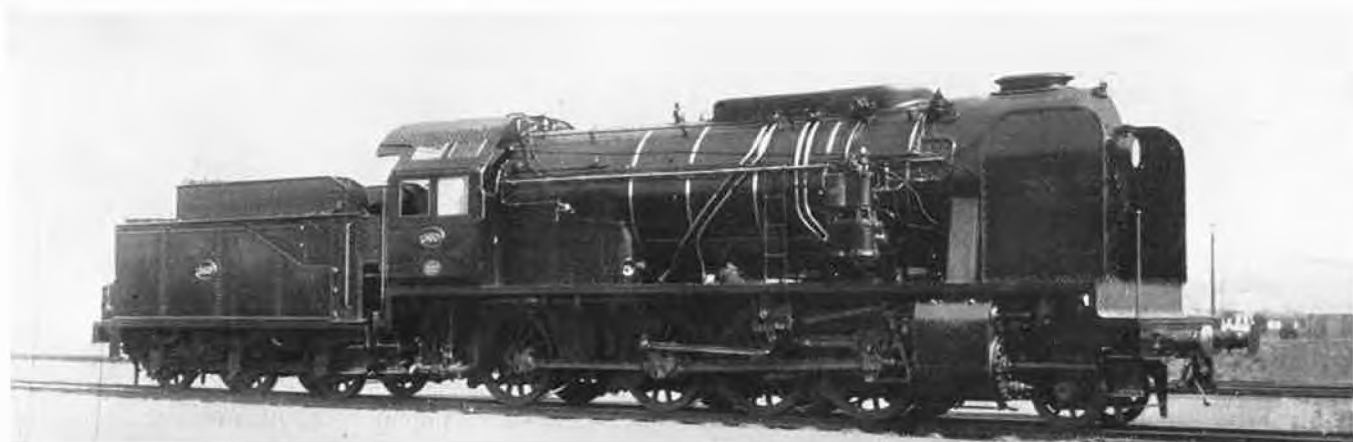
Consolidation (2-8-0) type goods engine for heavily graded lines
