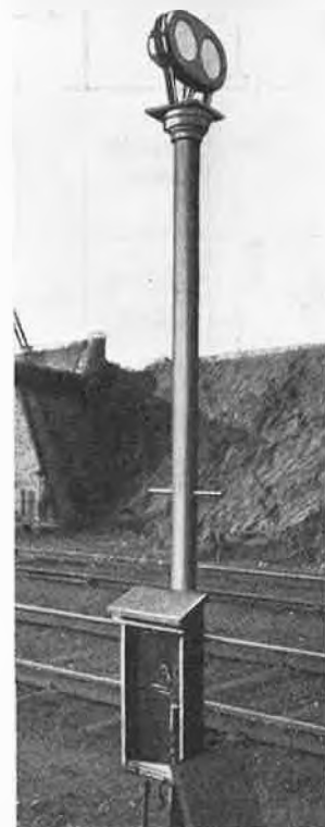
Fig. 2—A fog repeater installed on Brussels-Antwerp line in 1908
