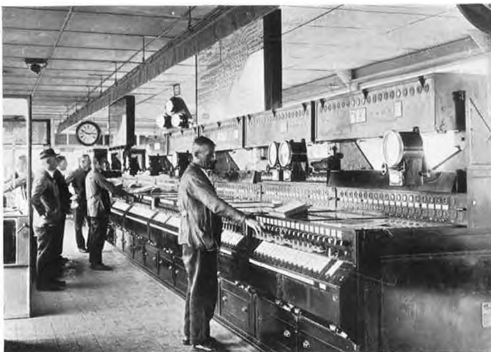
Fig. 20—Interior of new electric power signal cabin at Brussels Nord, A.C.E.C. system
